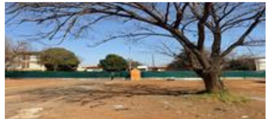
Figure 4 Bulk Earth work portion 1
