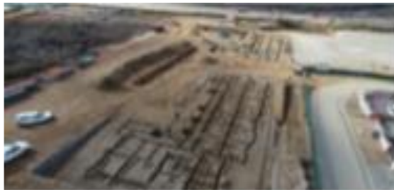
Figure 5 CLAYVILLE SITE CLEARING
